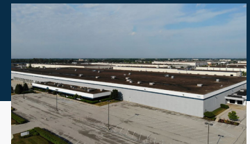
7520 Georgetown Rd Indianapolis, IN 424,849 SF | $29M
