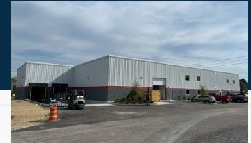
7098 Guion Road Indianapolis, IN 14,080 SF | $2.25M
