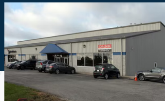
7050 Guion Road Indianapolis, IN 23,000 SF | $2.3M
